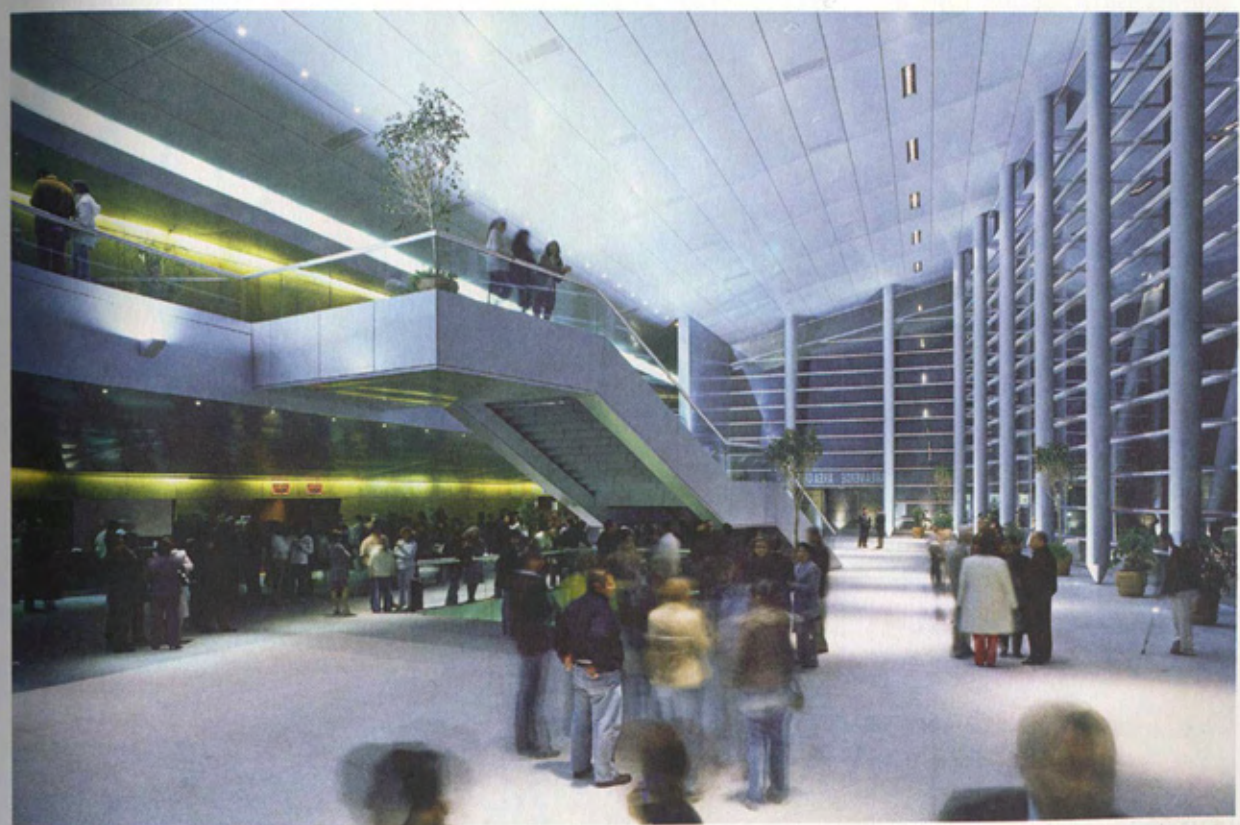
One of the main features is the cantilevered roof that houses an anchoring system for hundreds of glass and mirror sheets.
